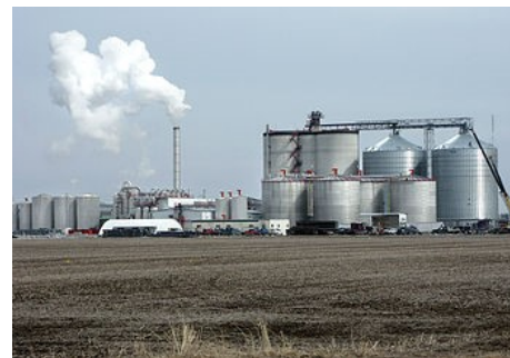
An ethanol fuel plant in West Burlington, Iowa.
