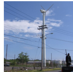
A wind turbine installation on I-95 in Fair Haven, Conn.
